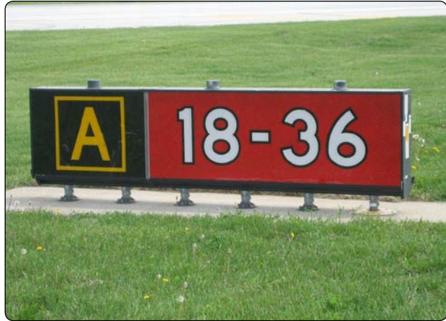
Figure 1-20. Runway holding position sign at a location other than the takeoff end of Runway 18-36 with collocated Taxiway Alpha location sign.
