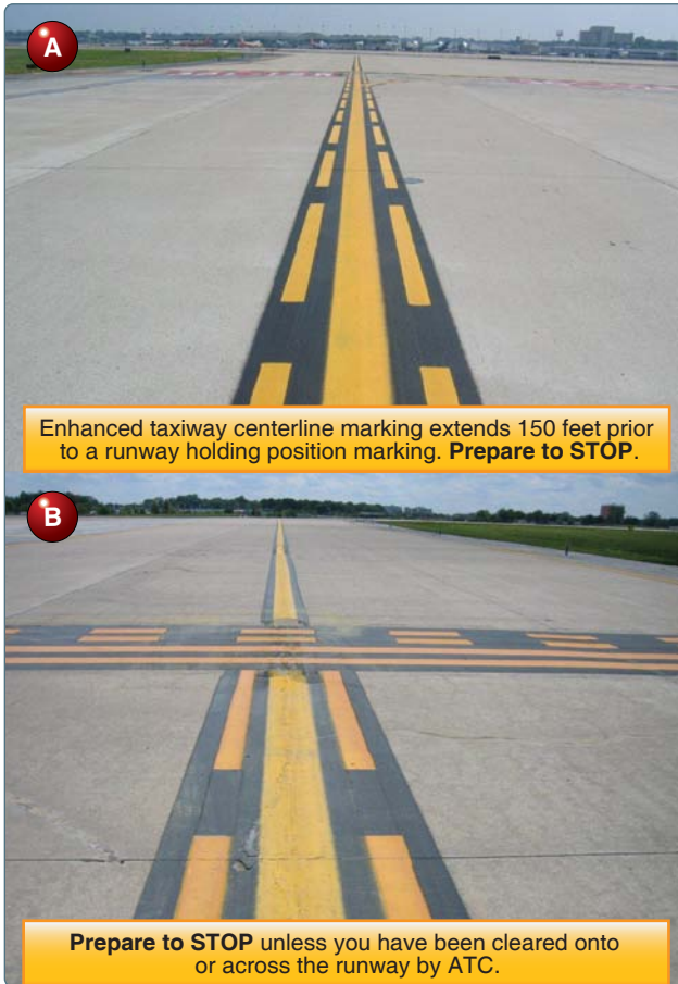
Figure 1-25. (A) Enhanced taxiway centerline marking. (B) Enhanced taxiway centerline marking and runway position marking.
