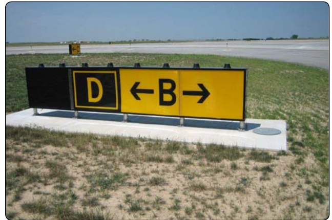
Figure 1-31. Taxiway Bravo direction sign with a collocated Taxiway Delta location sign. When the arrow on the direction sign indicates a turn, the sign is located prior to the intersection.
